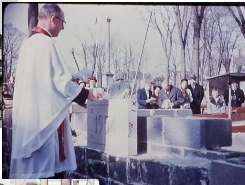
(below) The 1954 cornerstone is readied for placement.
