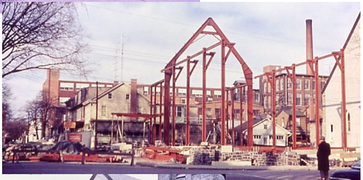
(right) The new building begins to take shape.
