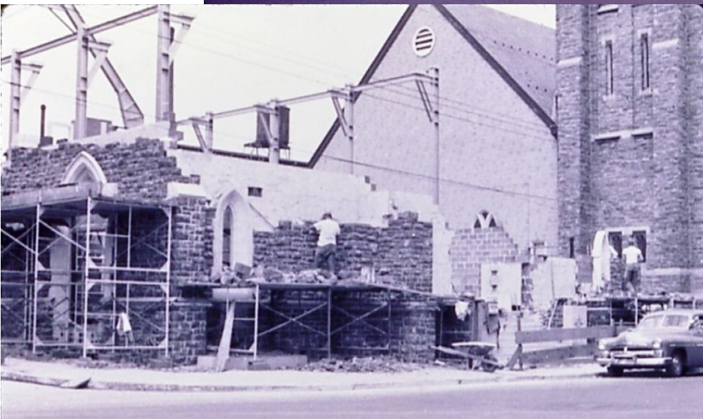
(left) The stonework slowly rising from sidewalk level.
